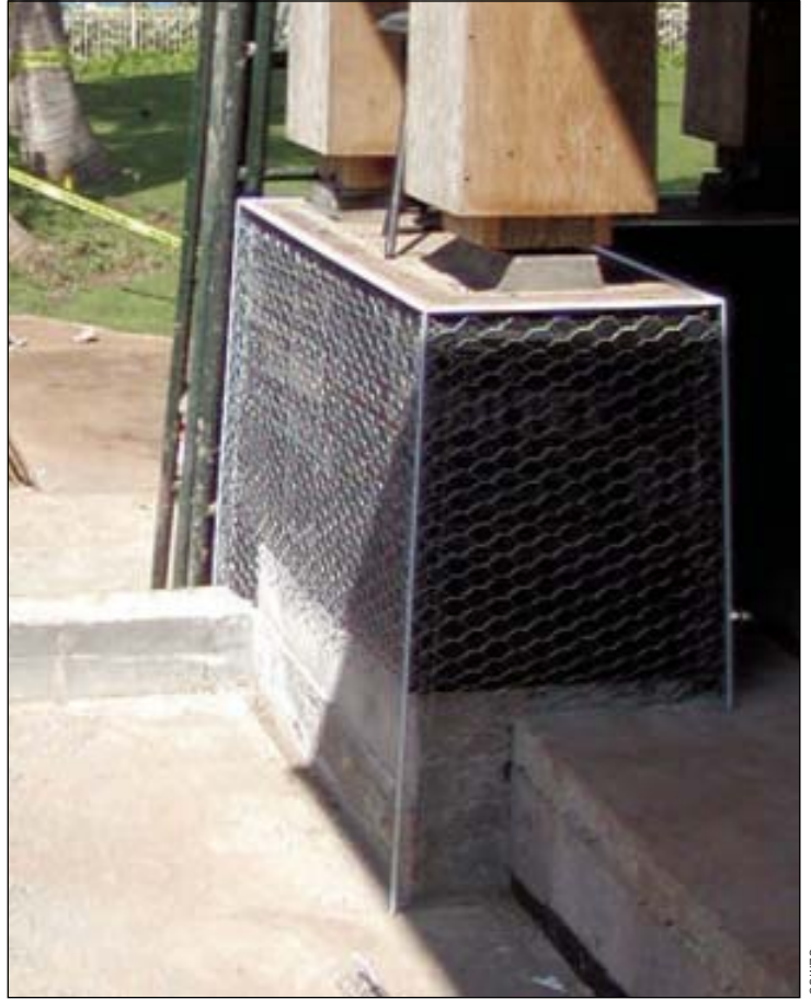
FIGURE 1. CORNER BEAD. To prevent stucco from popping off at outside corners, use corner bead. An alternative (not shown) is to round the corner, allowing the lath to poach out and provide plenty of room for stucco to key to the lath. The end result is a rounded corner that may not be compatible with all architectural styles.
