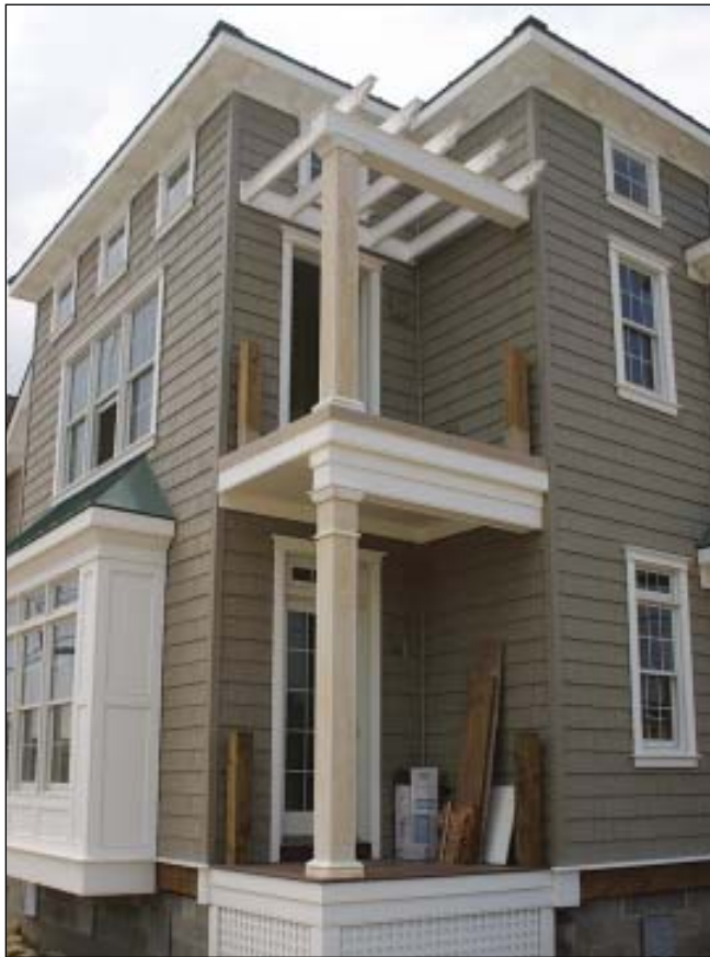
FIGURE 1. The column shown above is designed to carry an upper-story porch; details may vary slightly for columns that carry both an upper deck and a lower deck. However, the principles are the same for any porch/deck configuration, as detailed in the illustration on page 27: The exteriors are composed of layered, weather-tolerant, low-maintenance synthetic materials, while the inner structures are strengthened by reinforced masonry, engineered connectors, and treated wood.
