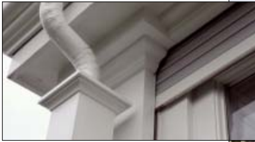
FIGURE 3. In the design for a renovated home on Nantucket Harbor, the authors specified roll-down shutters to shade and protect the sunroom windows and French doors facing the water. The shutters slide on tracks hidden behind the trim.
