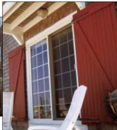
FIGURE 2. In the design of Nantucket's Harborside Cottages, the only waterfront condominium on the island, the authors called for custom board-and-batten exterior shutters to convey a traditional boathouse appearance to the individual units.
