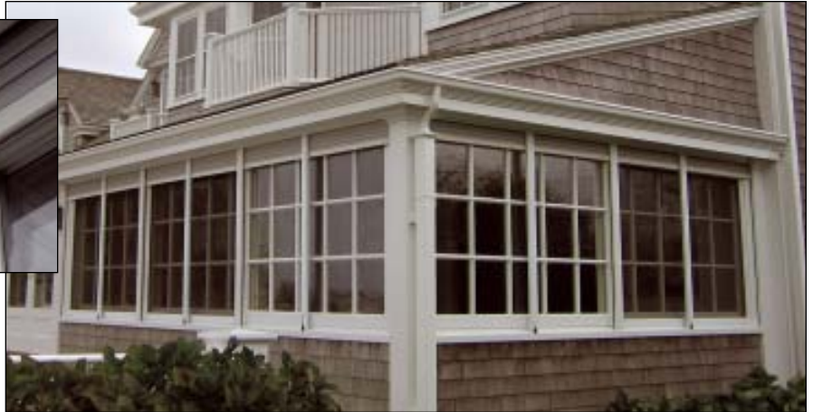
FIGURE 4. The authors incorporated the exterior-mounted box required for the rolling shutters into the design of the building cornice. Removable soffit panels provide access to the shutter for maintenance.
