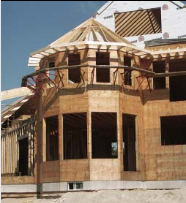
FIGURE 2. Using a pure geometric form helps maintain simplicity and symmetry in design massing, as well as in construction details such as roof framing.
