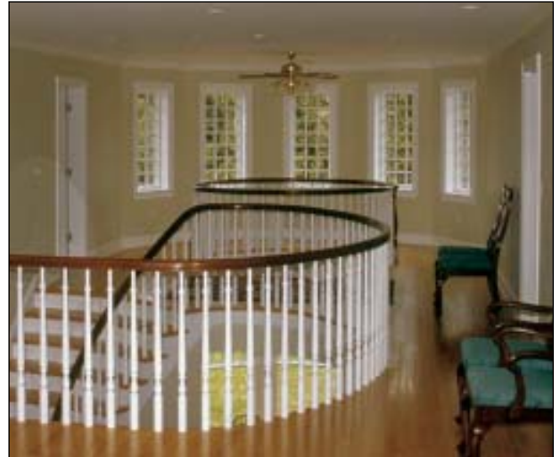
FIGURE 3. A figure with 12 or more sides can be adapted to a round exterior shape with curved horizontal furring. Inside, the windows bring in views, light, and air, and staying with a flat wall surface allows the use of simple mitered trim details (left). Upstairs (above), the curved, windowed wall opens up the end of a long hall space defined by structural walls.
