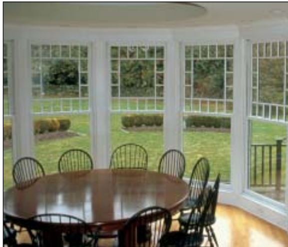
FIGURE 3. A figure with 12 or more sides can be adapted to a round exterior shape with curved horizontal furring. Inside, the windows bring in views, light, and air, and staying with a flat wall surface allows the use of simple mitered trim details (left). Upstairs (above), the curved, windowed wall opens up the end of a long hall space defined by structural walls.
