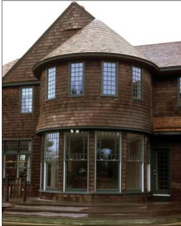
FIGURE 1. A multisided projecting room with windows adds interest to the elevation and brings in light while offering expansive views. The tower is a section of a duodecagon — a 12-sided figure that can be readily adapted to a circular form on the outside.
