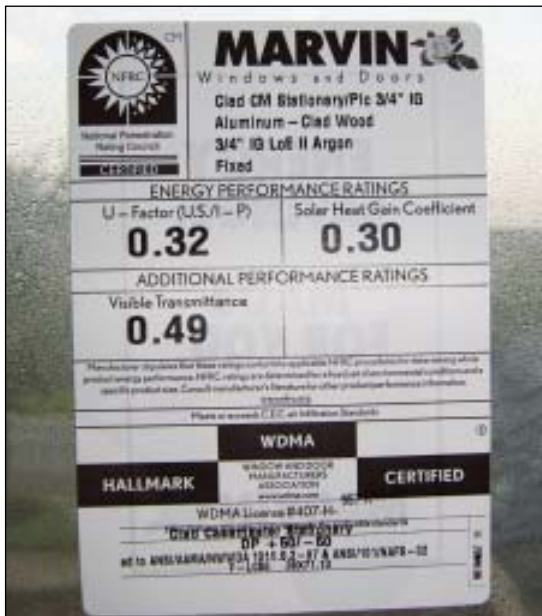
FIGURE 1. An NFRC label rates the basic energy performance of a window using two critical numbers: the U-factor, which measures heat flow, and the solar heat gain coefficient (SHGC), which measures the percentage of radiant heat energy that will pass through the window. For optimal performance in all climates, both numbers should be below 0.35.
