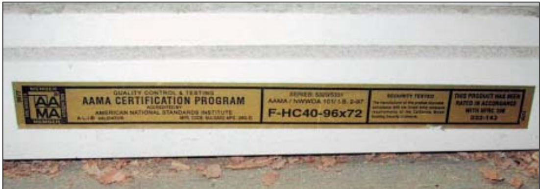
FIGURE 6. On this AAMA label, F-HC40-96x72 is the critical designation for this window. F is the product type (Fixed); HC is the performance class (Heavy Commercial); 40 is the performance grade (40 psf design pressure); and 96x72 is the maximum size tested (width x height).
