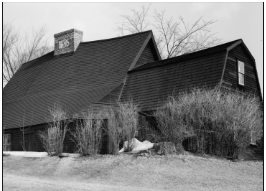
Considered the oldest wood-framed house in North America, the John Fairbanks house in Dedham, Mass., dates to 1636. The two gambrel additions were completed later, probably around 1668.
