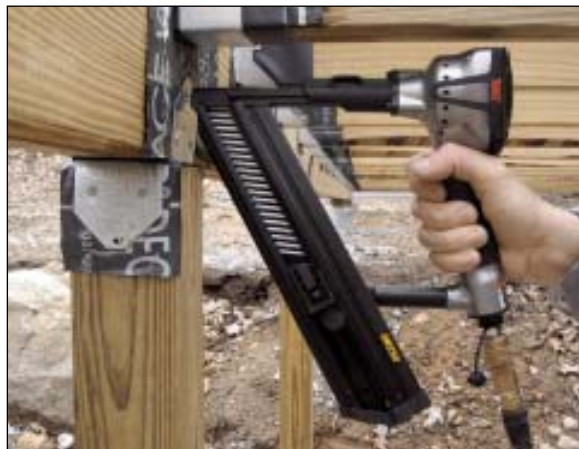
FIGURE 1. The big advantages of multi-blow hammers are safety and control: there's no chance of a ricochet off the hardware, and it's easy to seat the nail properly.
