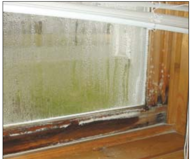
FIGURE 1. High indoor humidity levels, aggravated by a window blind that reduced the drying effect of air circulation, has created a condensation problem that has led to mold growth. In this case, the homeowner's lifestyle lies at the root of the problem, but it's not helped by an ordinary insulated window without warm-edge low-conductive glass.
