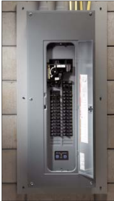
An integrated double-pole, double-throw transfer switch safely disconnects house circuits from the utility before connecting them to the generator, while maintaining a continuous ground for both power sources. The switch may be manual (above) or automatic (right).
