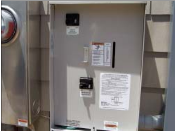
An integrated double-pole, double-throw transfer switch safely disconnects house circuits from the utility before connecting them to the generator, while maintaining a continuous ground for both power sources. The switch may be manual (above) or automatic (right).
