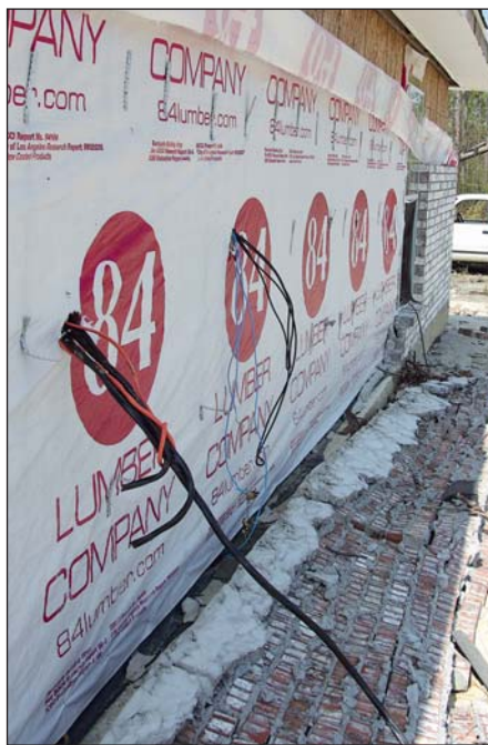
FIGURE 3. Hurricane Katrina's winds pulled a large section of brick off a Mississippi home (above left). Brick was also blown off a partially constructed wall (above); investigators found insufficient tie spacing, and noted that some ties (lower left) had been nailed to the wall, but not embedded into the mortar joints.
