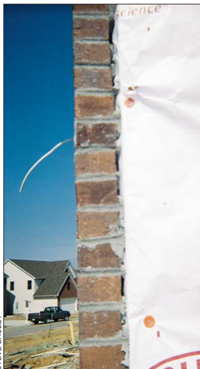
FIGURE 6. Good water management for walls requires an air space for water to drain down to the base of the wall, and an exit path for that water to flow to the outside. The brick at left has been laid without an adequate air space, making it likely that water will get trapped. Above is one way to provide an exit path for water: set natural-fiber rope into the mortar joints so that water can wick out. As the ropes decay over time, a clear drain path will open for the water.
