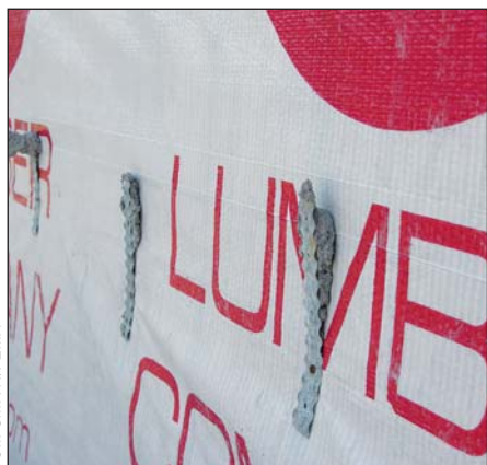
FIGURE 3. Hurricane Katrina's winds pulled a large section of brick off a Mississippi home (above left). Brick was also blown off a partially constructed wall (above); investigators found insufficient tie spacing, and noted that some ties (lower left) had been nailed to the wall, but not embedded into the mortar joints.
