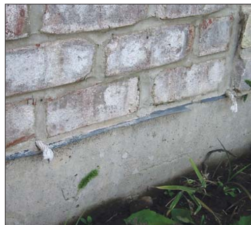
FIGURE 6. Good water management for walls requires an air space for water to drain down to the base of the wall, and an exit path for that water to flow to the outside. The brick at left has been laid without an adequate air space, making it likely that water will get trapped. Above is one way to provide an exit path for water: set natural-fiber rope into the mortar joints so that water can wick out. As the ropes decay over time, a clear drain path will open for the water.
