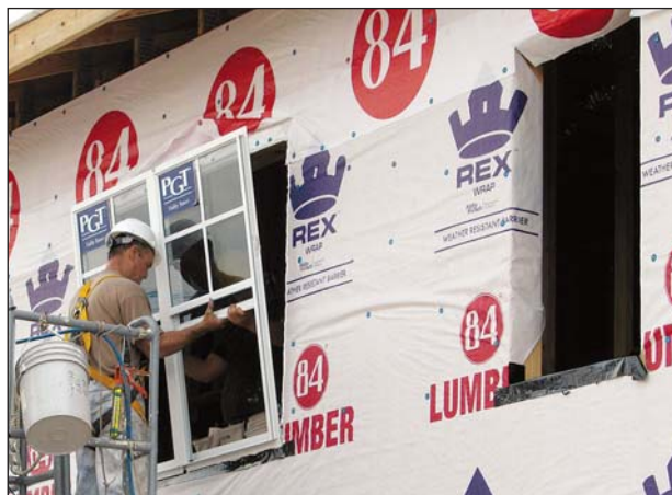
FIGURE 6. The WRB can be installed before or after the window, depending on contractor preference. If put on afterward, the sill must be lined with a water-resistant barrier before the window gets hung. Although few manufacturers provide clear guidance on flashing, appropriate systems are documented in industry standards.
