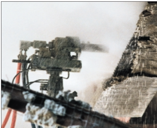
Above: Twelve-inch concrete is being cut with a 40,000-psi water jet that has fine garnet aggregate fed into the water stream at the nozzle. The nozzle is guided on a rail.
