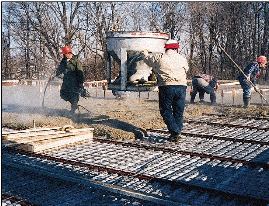
Figure 1. Workers place concrete on a steel-joist floor.
