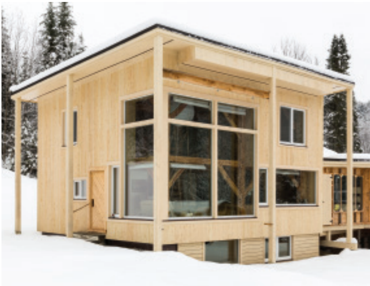
The Whitchurch "in-law" annex in Vermont has an unvented flat roof that relies on a ProClima Intello variable-permeability membrane to limit moisture accumulation in winter and allow drying in summer.
