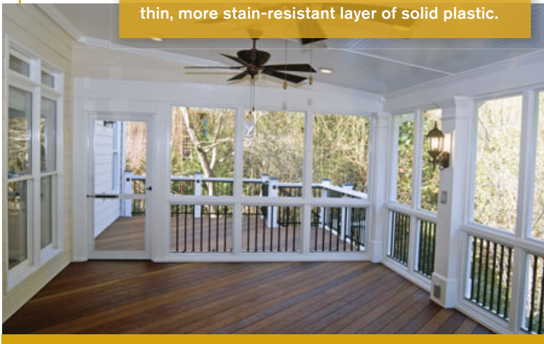
Figure 2. Capstock decking, such as Fiberon's Horizon, is composite material covered with a thin, more stain-resistant layer of solid plastic.
