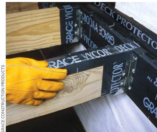
Figure 2. Peel-and-stick membranes can be used to isolate metal from wood preservatives, thereby reducing corrosion. When protected from long-term exposure to the sun, they may even be used in place of rigid flashings in some jurisdictions.
