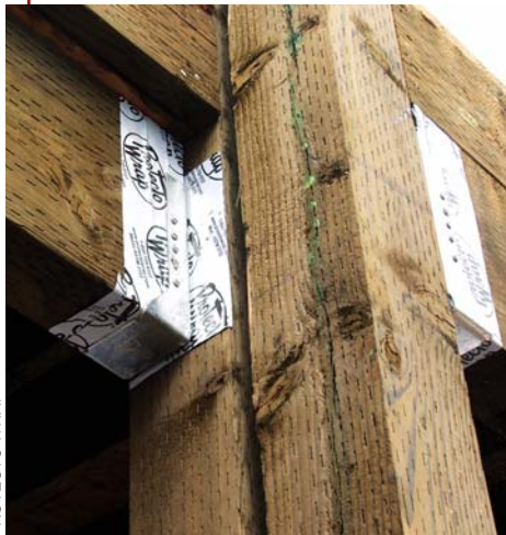
Figure 3. Galvanized framing hardware may also be prone to accelerated corrosion from some preservatives. Isolating it with peel-and-stick may increase the galvanization's lifespan.
