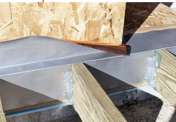
Figure 4. Installed with the copper face to the treated lumber and the polymer face out, hybrids can both flash and isolate galvanized hardware.
