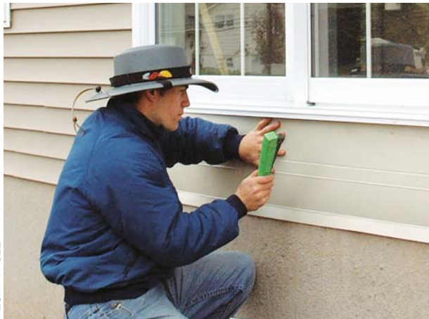
Figure 5. Rigid PVC flashings have no risk of corrosion, can be exposed to the sun, and may be bent on a sheet-metal brake or along factory-made creases.
