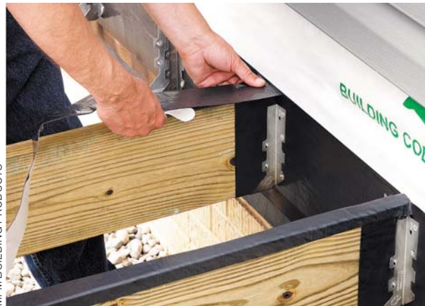
Figure 6. Flashing is not just for the ledger. Particularly in the West, where wood species used for treated lumber don't absorb preservatives that well, flashing the tops of joists and beams can keep out water and reduce the potential for rot.
