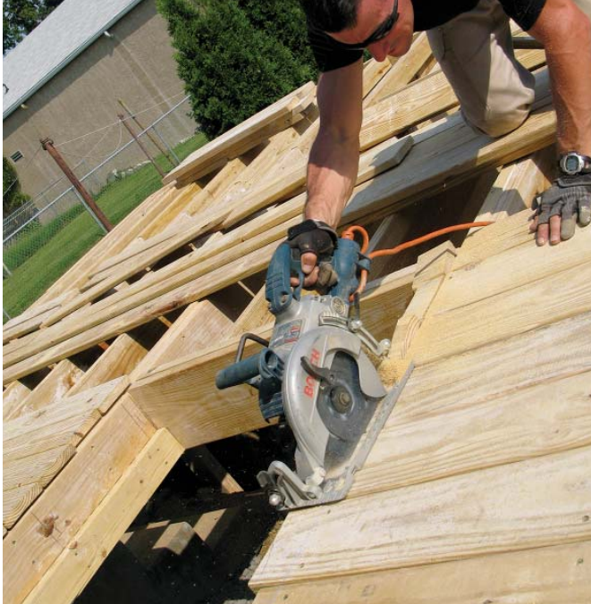
Figure 2. TimberSil is southern yellow pine that has been infused with glass. The maker, Timber Treatment Technologies, claims that its product offers greater span ratings than standard treated southern pine. It's also much harder — about as hard as hickory. The company says the product is extremely “green.” (703/644-0991, www.timbersilwood.com )
