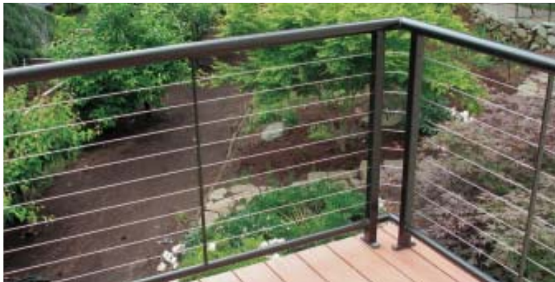
Figure 8. Code requirements for railing combustibility are sketchy and subject to interpretation. One sure approach is a noncombustible system made from metal.
