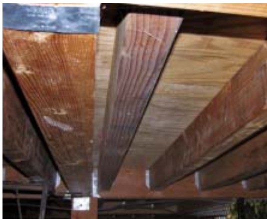
Figure 4. Heavy timber is one way to frame a fire-resistant deck. The larger the lumber, the harder it is to ignite, and the less intense the heat it contributes. National codes specify a minimum of 4x6 joists, 6x10 beams, and 8x8 posts.
