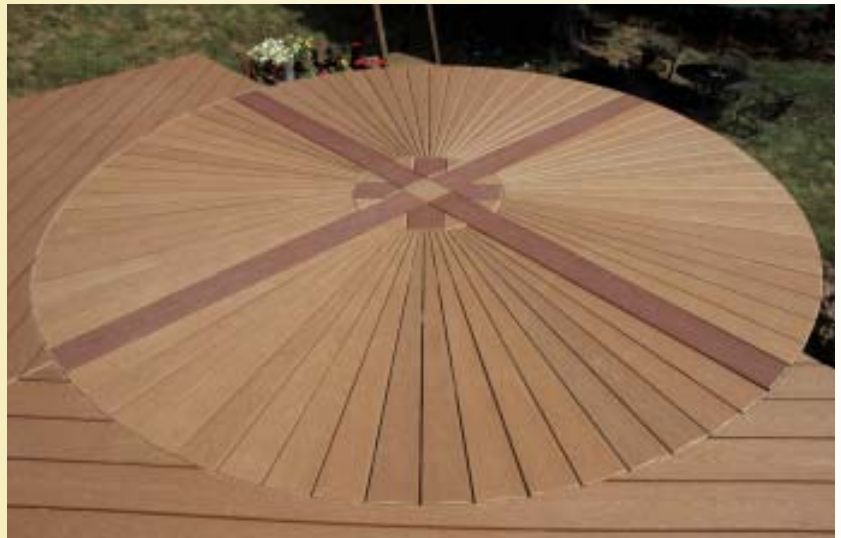
Figure 8. Wedge-shaped decking boards make up the fan pattern. Dividing the circle into quadrants with a cross pattern facilitates installation and creates a distinctive motif.
