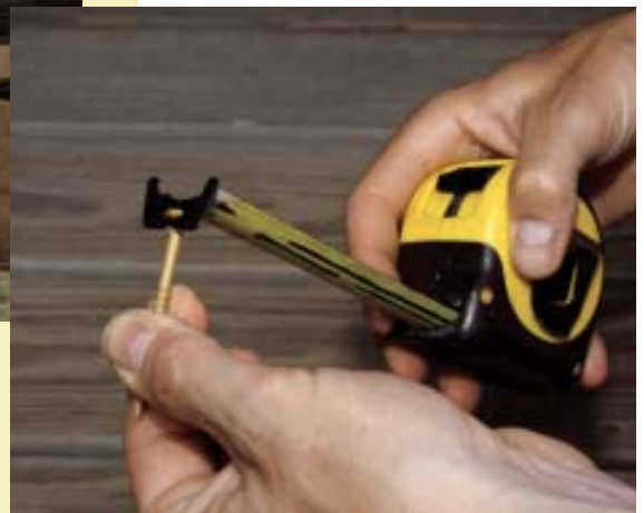
Figure 6. Curved shims are screwed to the band board to support a curved fascia (above). A tape measure hooked on the head of a screw (right) set at the center point is used to lay out the curve on one piece of 2-by, which is cut out carefully and used as a template for the rest.
