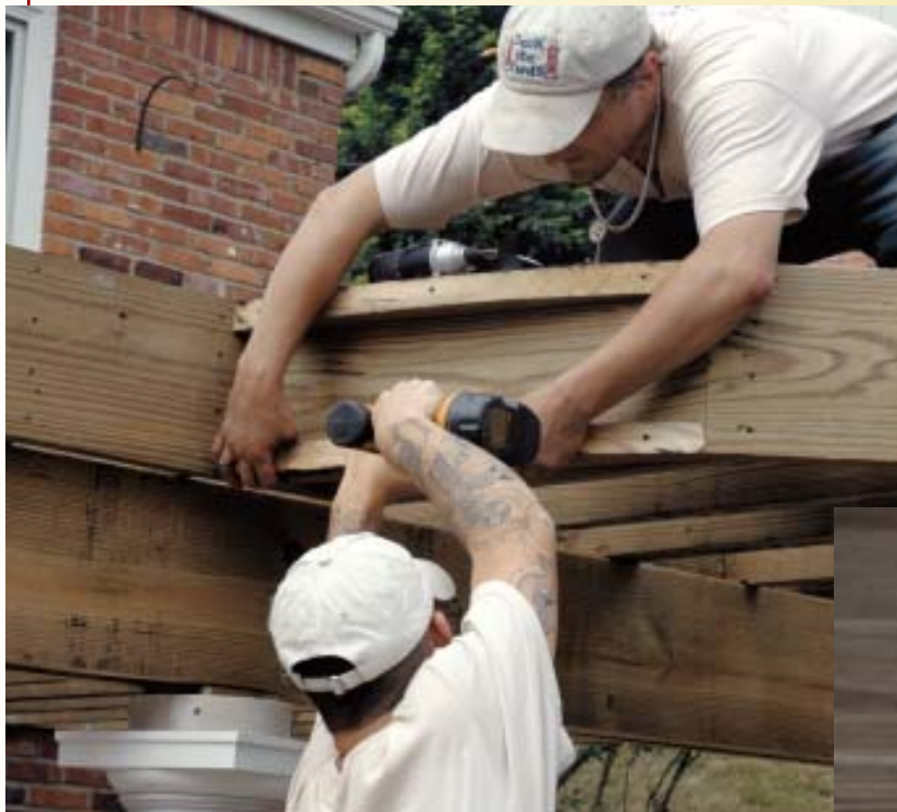
Figure 6. Curved shims are screwed to the band board to support a curved fascia (above). A tape measure hooked on the head of a screw (right) set at the center point is used to lay out the curve on one piece of 2-by, which is cut out carefully and used as a template for the rest.
