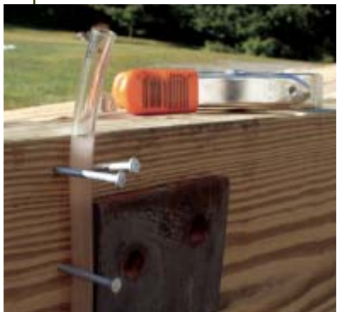
Figure 3. There must be 50 ways to hold your level, but nails and clamps will do the trick. The key is to hold the end in a way that permits it to be moved for fine-tuning, but that doesn't close off the tube.
