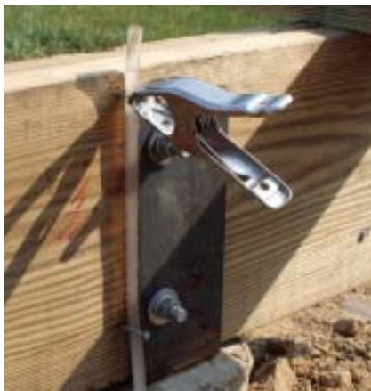
Figure 3. There must be 50 ways to hold your level, but nails and clamps will do the trick. The key is to hold the end in a way that permits it to be moved for fine-tuning, but that doesn't close off the tube.
