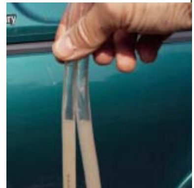
Figure 1. As long as the rules of physics don't change, water levels will work. It doesn't matter if the two ends of the tubing are right next to each other, or a hundred feet away. Water seeking its own level provides level benchmarks for the deck builder's convenience.
