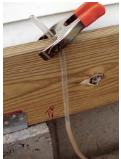
Figure 3. There must be 50 ways to hold your level, but nails and clamps will do the trick. The key is to hold the end in a way that permits it to be moved for fine-tuning, but that doesn't close off the tube.
