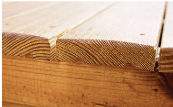
Figure 1. The winner of NADRA's 2011 Deck Competition, Tailor Decks, specifies all-sapwood 2-inch KDAT lumber that's milled with a crowned top, beveled sides, and kerfs on the bottom.
