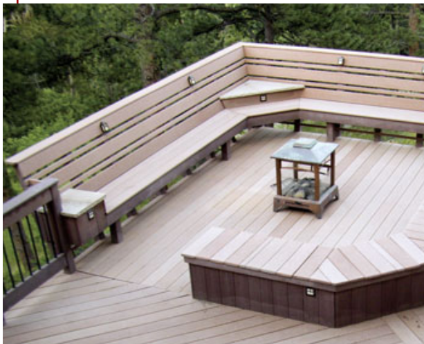
Figure 1. Although code compliant when built under the 2003 IRC, the bench seat at the edge of the second-level deck shown here would not comply with the 2009 IRC because its back extends only 24 inches above the seating surface.
