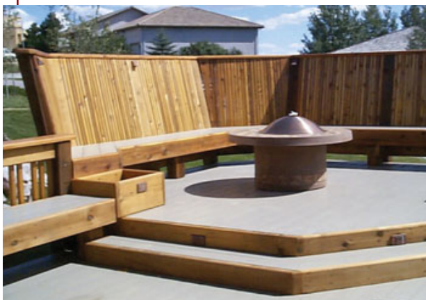
Figure 2. The combination guard and bench in this photo was constructed to function as a privacy wall; the back would be compliant with the new IRC requirement that guards behind adjacent fixed seating be at least 36 inches higher than the seat's surface.
