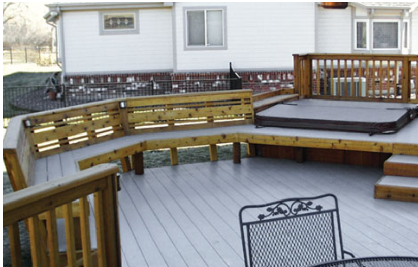
Figure 3. In this design, the deck surface surrounding the hot tub smoothly connects to the bench at the left. Only in designs similar to this one should the bench seat be considered a “walking surface.”
