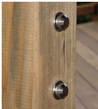
Figure 5. One upgrade the author chooses is stainless steel caps, rather than plastic ones, to conceal the cable ends.
