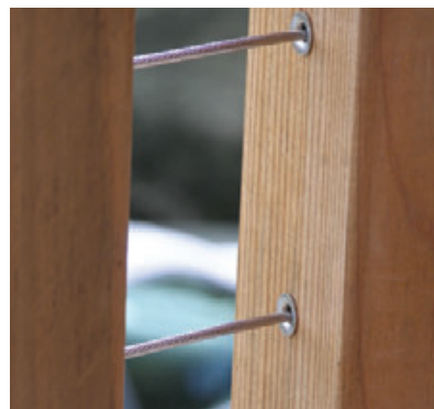
Figure 2. Where cables turn a corner or change angle for a stair, liners are used to prevent the cable from wearing down the wood posts.
