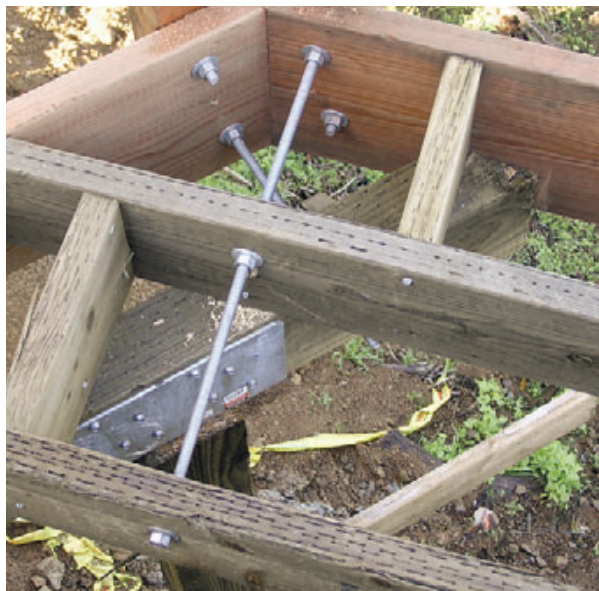
Figure 6. Posts are anchored to the framing with 1/2-inch galvanized threaded rod.
