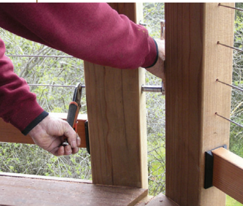
Figure 15. Go back to where you started and finish tensioning the cables by tightening the nuts.
