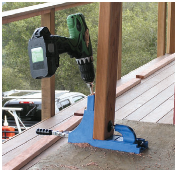
Figure 7. Sub-rails are attached to the posts with pocket screws.
