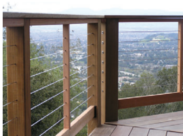
Figure 3. Even though cables are tensioned, they can sag mid-span. A lighter-duty member is used between the posts to maintain cable spacing.
