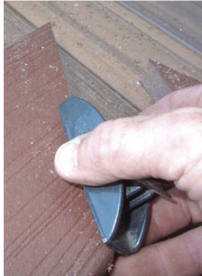
Figure 19. Bevel abutting edges with a few passes of a block plane.
