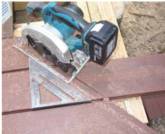
Figure 17. Use a layout square and a circular saw to miter corners after installation.
