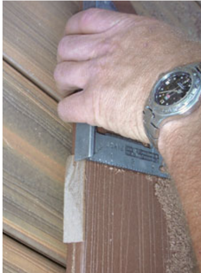
Figure 18. A piece of paper or cardboard between a square and the board is a quick and consistent way to make minor angle adjustments.
