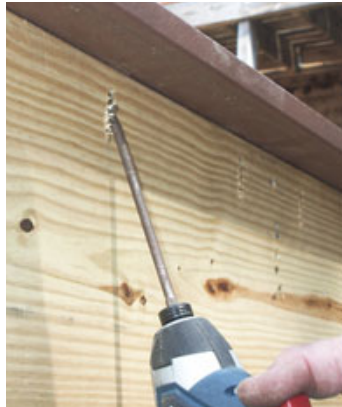
Figure 15. Pocket screws from below are a slick way to hide fasteners at the ledger and rim joists.
