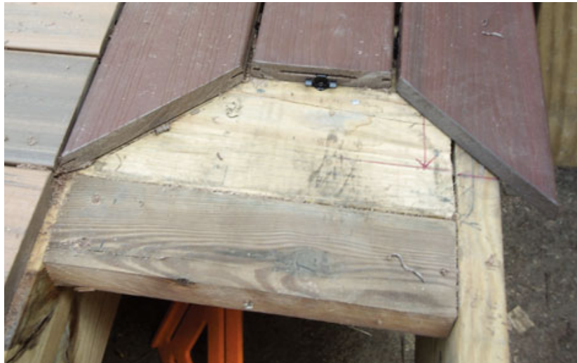
Figure 21. A returned miter joins the outer boards of a picture frame.
