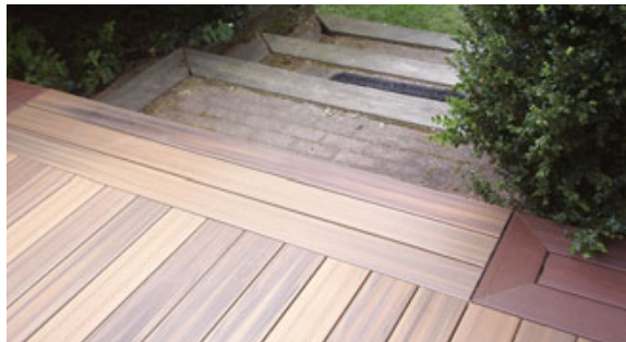
Figure 6. Wider borders have a greater visual impact, but the deck has to be large enough for the border to be in proportion.
