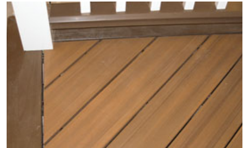
Figure 5. Running the field decking on a diagonal emphasizes the border.
