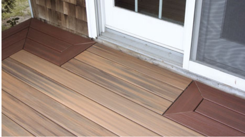
Figure 14. Aligning a border with a feature such as a door not only looks sharp, it helps guide traffic.
