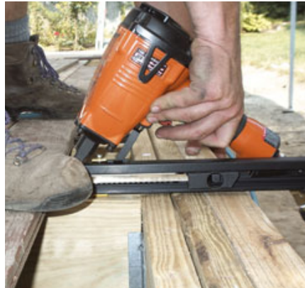
Figure 16. Hidden fastener nailers speed installation but can be awkward to use.
