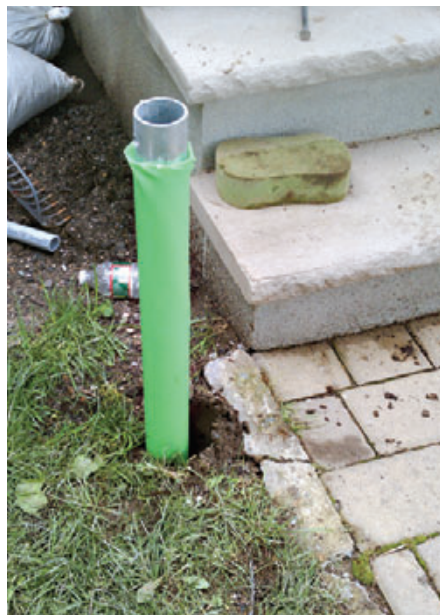
Figure 12. Because helical piles don't disturb the ground much, they can be installed alongside existing landscape features.
