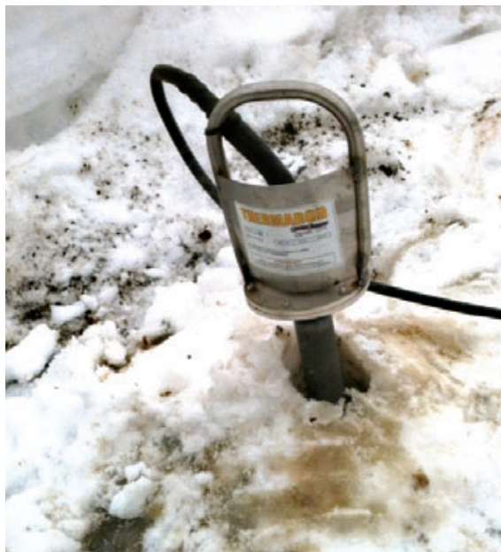
Figure 10. Driving a helical pile in frozen ground begins with inserting a proprietary heating rod in a hole drilled with a rotary hammer (above). Once the ground is warmed, the pile is driven normally (right).
