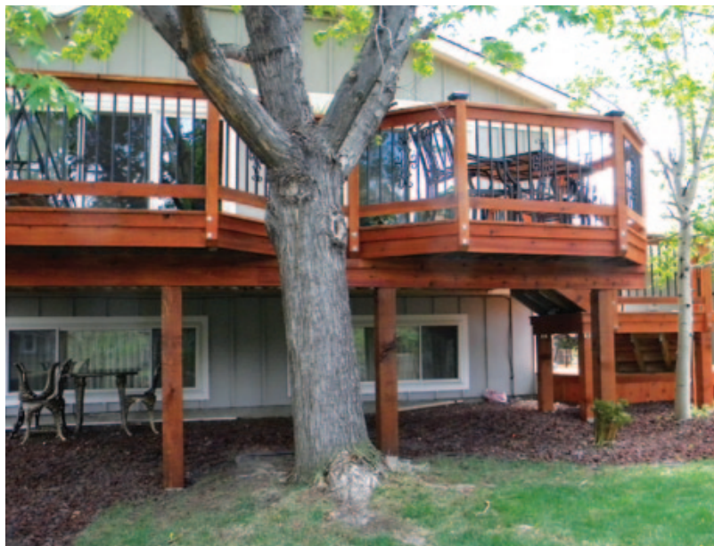
Figure 12. It's simpler and cheaper to make support columns and railing posts from wood (top). Once everything is wrapped with finish materials, it's impossible to tell what the underlying material is (bottom).
