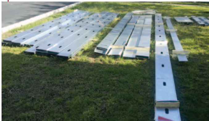
Figure 2. The author buys steel framing members pre-cut to the exact length needed.
