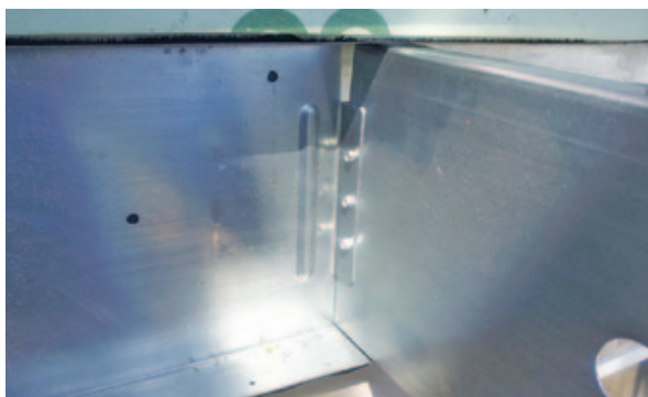
Figure 6. Ledger and rim track is available with tabs punched on standard framing layouts (above). The joists are screwed to these tabs (right).
