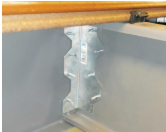
Figure 5. Some steel framing systems require the use of framing hardware to make connections.
