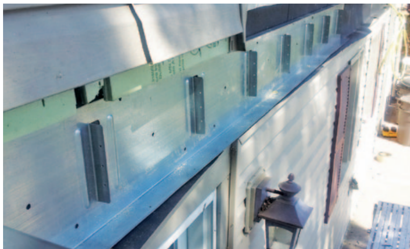
Figure 6. Ledger and rim track is available with tabs punched on standard framing layouts (above). The joists are screwed to these tabs (right).
