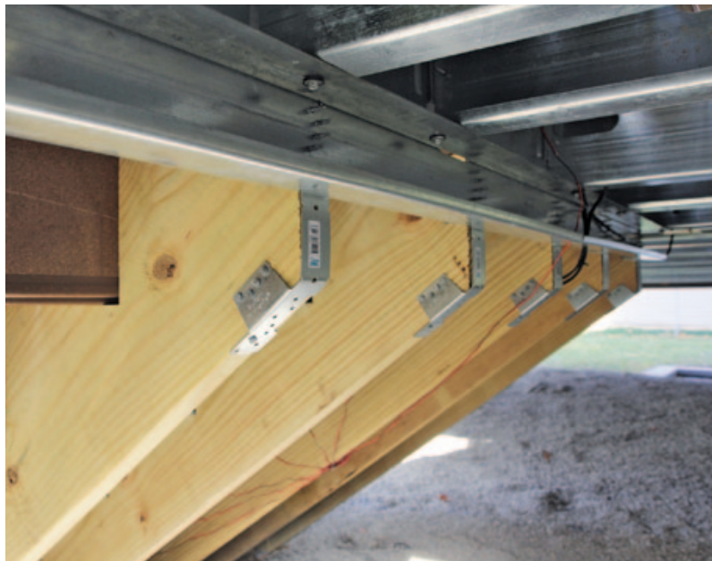
Figure 15. Stair stringers are typically made of wood, which is more economical and easier to wrap with finish materials.
