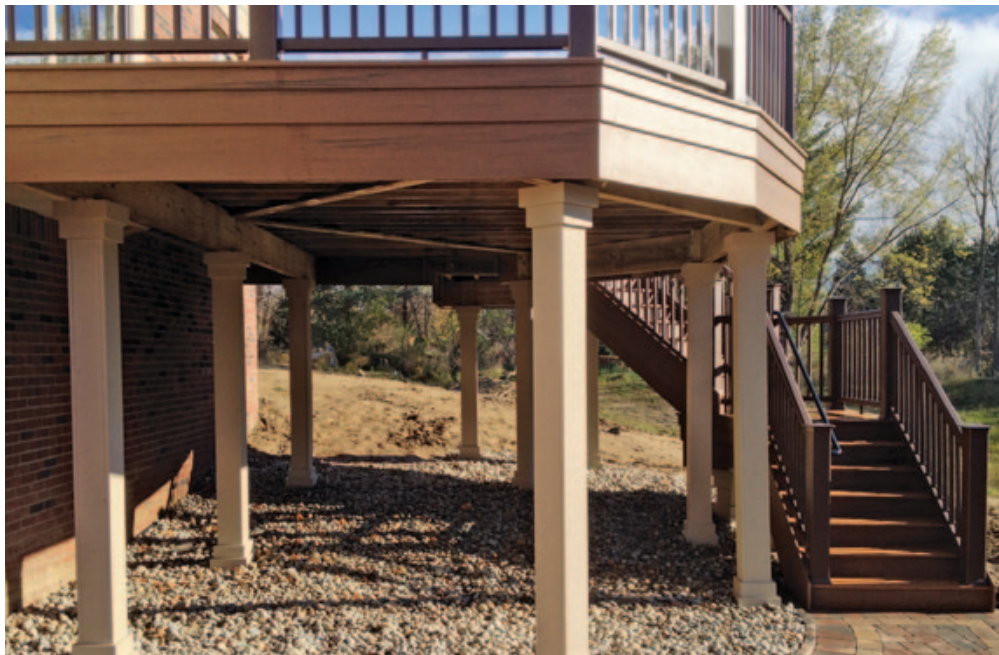
Figure 8. The author's "triple stacked" fascia extends just below the bottom of the support beam, concealing all the horizontal framing.
