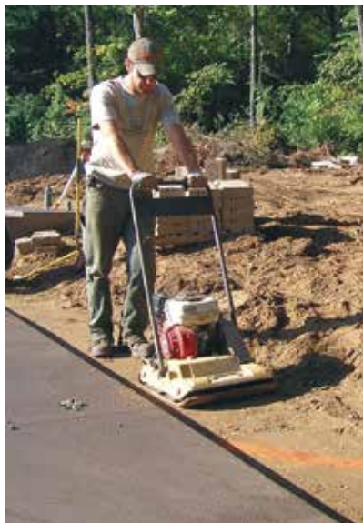
Figure 4. Segmental retaining walls don't require a concrete footing but do require a solid base of compacted crushed rock (below). Some manufacturers recommend adding a layer of coarse sand to make leveling the first course of block easier (bottom).
