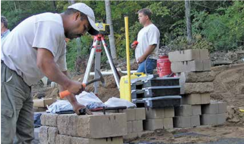
Figure 1. Some manufacturers use pins to align the blocks in their segmental retaining walls. Versa-Lok's pin system (left) ensures that each course has a 3/4-inch setback, giving the wall face an angle of about 7 degrees away from vertical.
