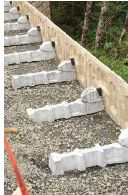
Figure 1. Some manufacturers use pins to align the blocks in their segmental retaining walls. Versa-Lok's pin system (left) ensures that each course has a 3/4-inch setback, giving the wall face an angle of about 7 degrees away from vertical.
