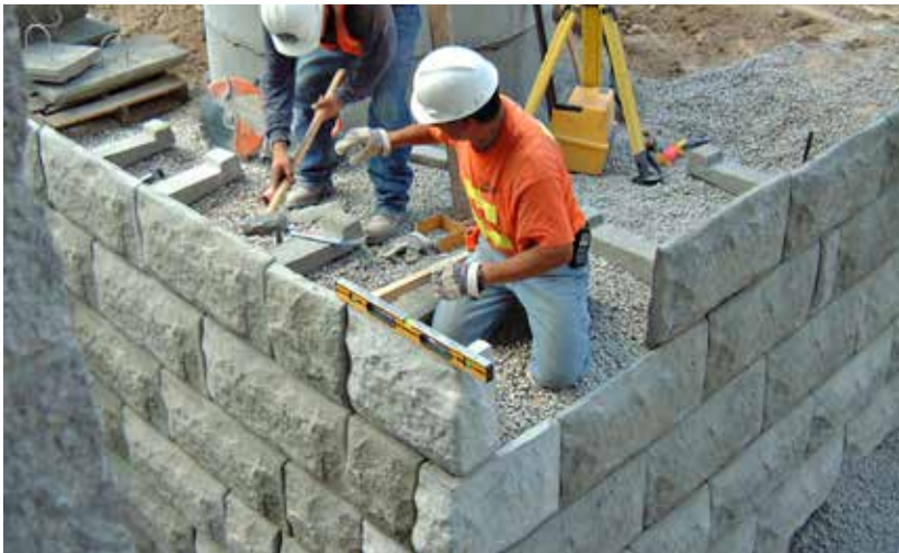
Figure 2. In Lock+Load's retaining wall system (above and right), face pieces are attached to separate anchoring components called counterforts. The counterforts work like geogrid fabric, anchoring each panel to the soil mass behind the wall.
