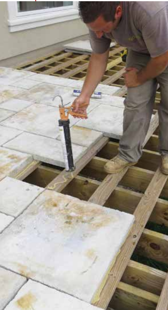
Figure 6. Paver installation goes quickly. Working from a CAD-generated pattern, workers apply landscaping stone adhesive to the sleepers (left), then fit the pavers into place (above). A 1/4-inch gap between the ungrouted pavers is critical for drainage.
