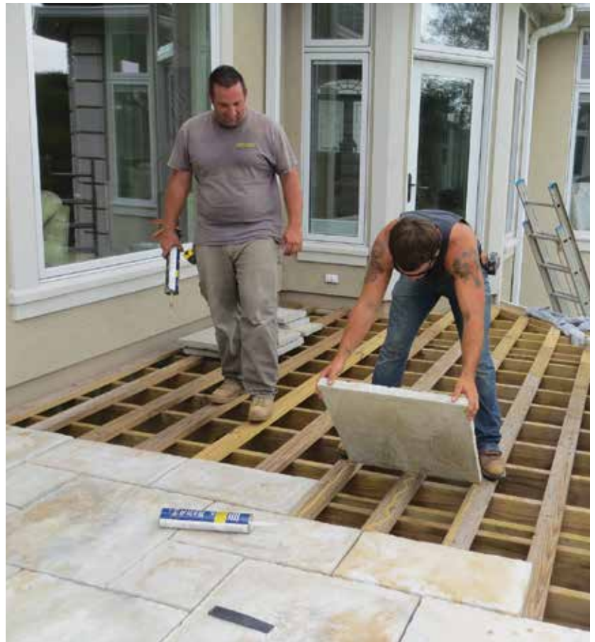
Figure 6. Paver installation goes quickly. Working from a CAD-generated pattern, workers apply landscaping stone adhesive to the sleepers (left), then fit the pavers into place (above). A 1/4-inch gap between the ungrouted pavers is critical for drainage.
