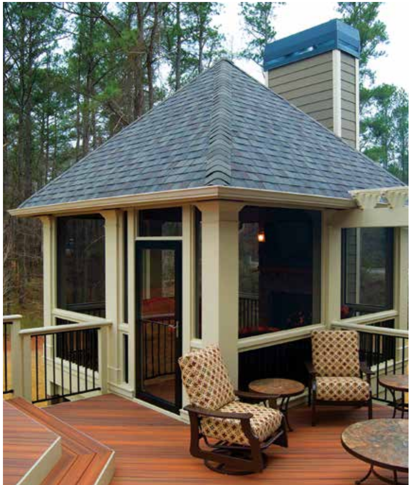
Figure 7. Hip roof framing, as for this detached porch (above), is more complicated than shed or gable roof framing, but when well-executed it can provide a dramatic vaulted ceiling (below).
