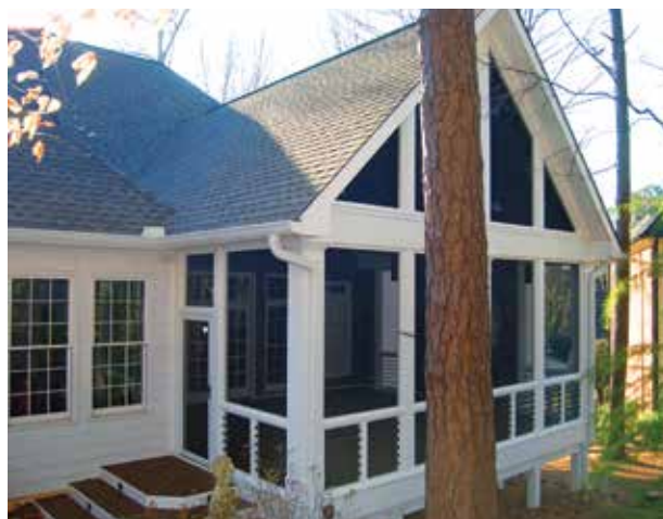
Figure 1. This home's full two-story wall design and small upper-floor windows allow a simple wall tie-in for the porch addition's gable roof (above left). Roof tie-ins involve more complex framing (above right), but are often needed on single-story structures where more interior porch volume is desired.
