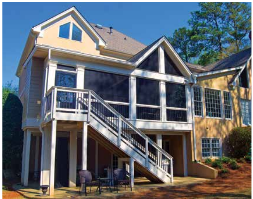
Figure 4. Shed and gable roofs can be combined on a porch. When designing an addition with a gable roof, match the pitch of any existing gables.
