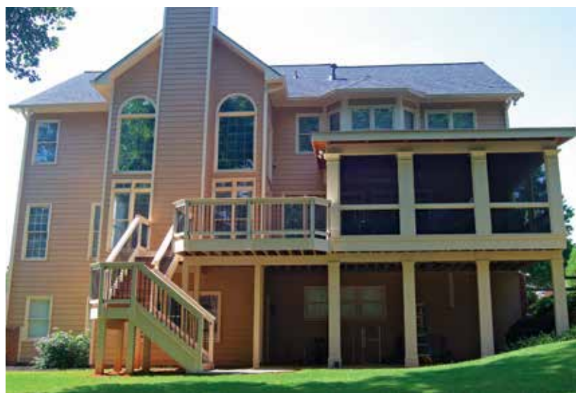
Figure 2. A shed style was the best solution for this porch roof because of restrictions placed by the existing second-story windows. It would also have been difficult to match the pitch of the existing gable roof next to the porch.
