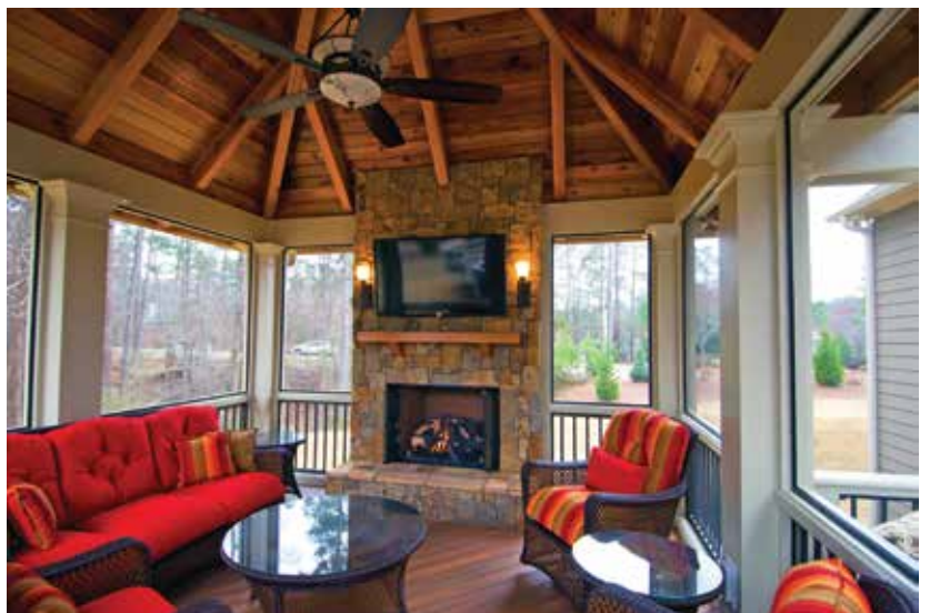
Figure 7. Hip roof framing, as for this detached porch (above), is more complicated than shed or gable roof framing, but when well-executed it can provide a dramatic vaulted ceiling (below).
