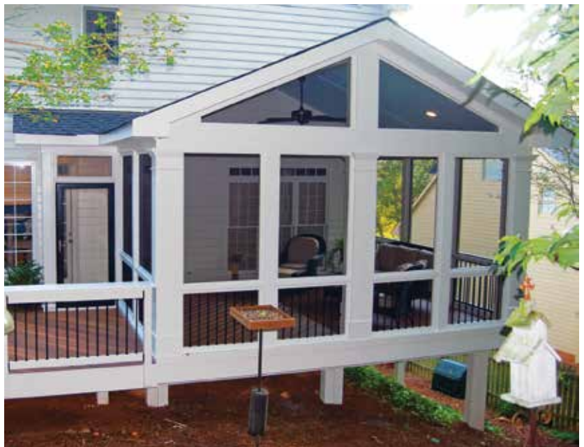
Figure 6. A small extension off this screened porch contains a captured doorway leading out onto the adjacent deck.
