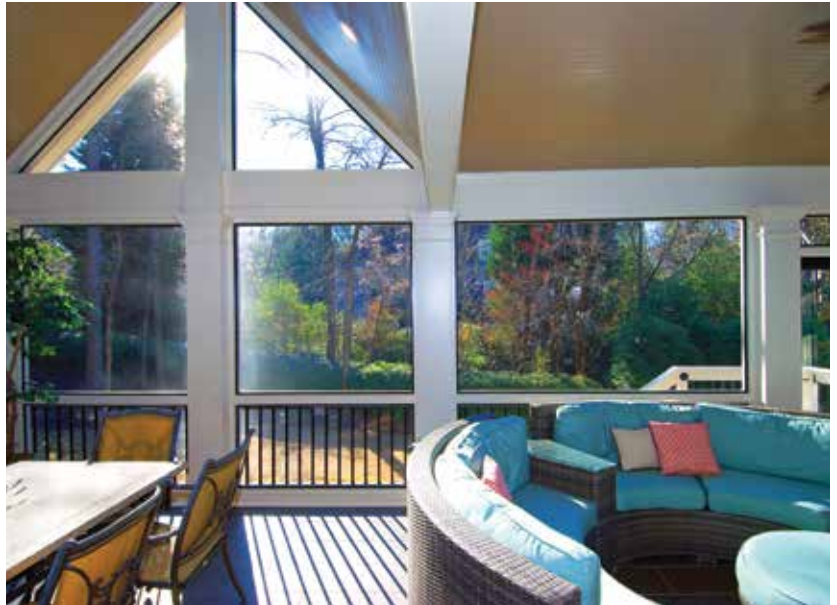
Figure 5. The framing for the gable and shed roof sections of the porch help define interior areas.
