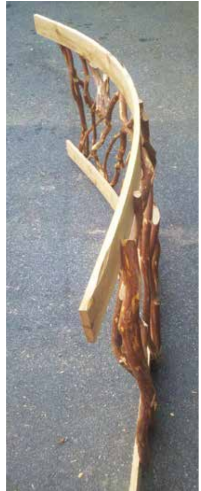
Figure 6. When a rail section is installed, a second pair of curved 1x4 rails and a horizontal 2-by top rail are added to complete the assembly.
