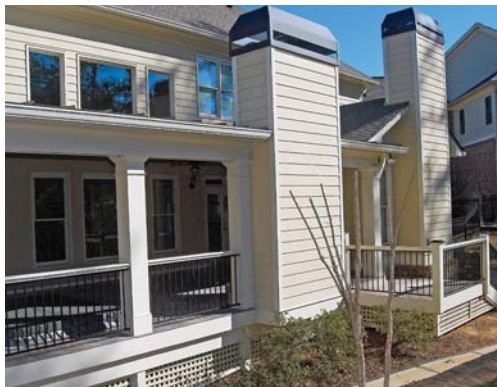
Figure 5. Because the top of the flue must be 2 feet above any part of the building that's within 10 feet, the location of the fireplace affects the flue's required height.
