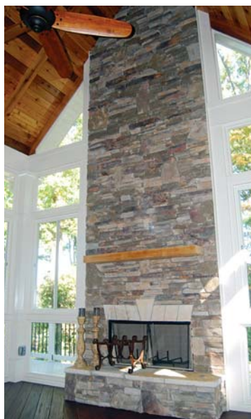
Figure 4. Particularly when paired with cathedral ceilings, end-wall fireplaces can make a dramatic, if expensive, statement.
