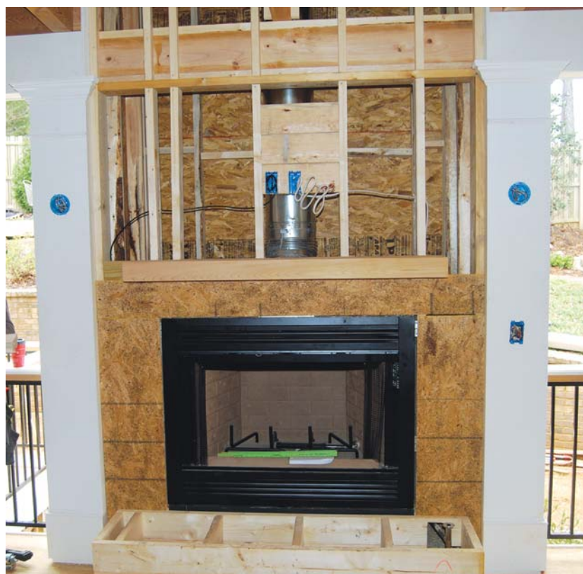
Figure 1. So-called zero-clearance fireplaces do in fact require some clearance to combustibles but so little that wood-framed chases are typical.
