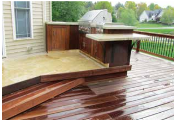
Angles make a space appear larger and more dynamic and can be used to create a nook that doesn't interfere with traffic flow. Note that the deck and patio surfaces have been "flip-flopped" on this project, which features Brentwood stone countertops that look like petrified wood, a travertine terrace, and cumaru decking.
