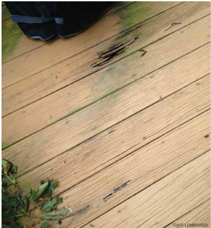
Figure 2. The same 5/4x6 ACQ stock that was used for the cap rail in the top photo was used for the decking, which also needed replacement.
