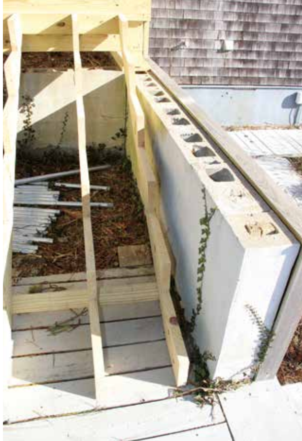
Figure 6. Check your lumber's end tag or ink mark to avoid inadvertently cutting stair stringers from PT stock that is only rated for above-ground use, and treat all cuts with copper naphthenate.
