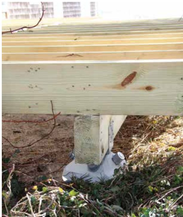
Figure 7. Ground-contact lumber should always be used for deck joists, beams, and other framing that is in close proximity to the ground.
