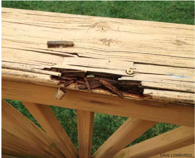
Figure 1. This deck was built in the mid-Atlantic area in 2005 using ACQ-lumber treated for above-ground use. The 5/4x6 cap rail shows clear signs of premature rot.
