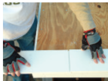
Figure 5. Longer lengths of PVC trim require a movement joint, which the author creates by first cutting a matching shiplap profile on the end of each board with a router (top). It's best to place a shiplap movement joint in an unobtrusive location, as the joint will be visible in cooler weather when the boards contract. Some builders fill the gap with sealant, but this step isn't necessary; the joint itself will block most moisture from penetrating to the substrate (above).
