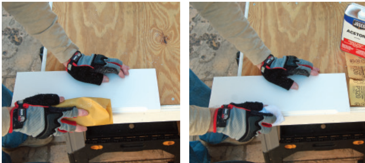
Figure 6. After cutting or routing PVC trim, the author gives the cut a light sanding with 320-grit paper (above left). After sanding, wiping the cut down with acetone (above right) causes a chemical reaction in the PVC that closes up the cells and prevents the cut edge from trapping dirt.
