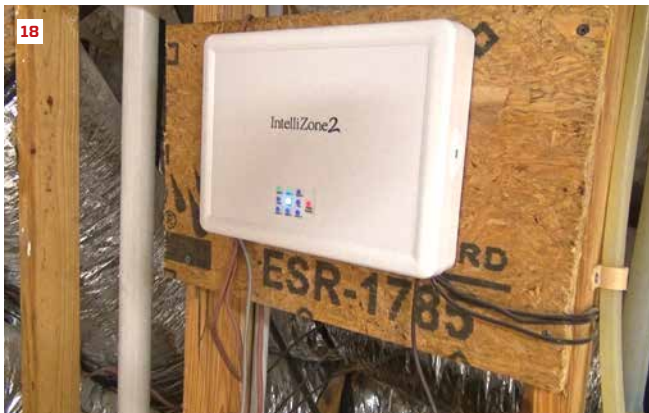
A preapplied paper ruler helps foam installers and inspectors verify application thickness (16). In this high-end system in an insulated attic, three zone supply ducts coming out of a distribution box are equipped with motor-controlled dampers (17); illuminated LEDs on the control device indicate which zones are active (18). Heat from the geothermal system also preheats hot water (19).
