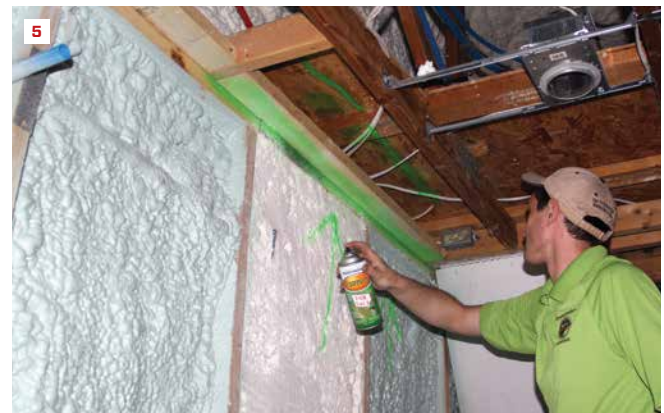
Technician Jack Hogan zeros the electronic manometer before the blower-door test (3). Hogan points out an air leak near the patio door (4). Hovis marks a gap in the foam insulation for correction by the foam crew (5).
