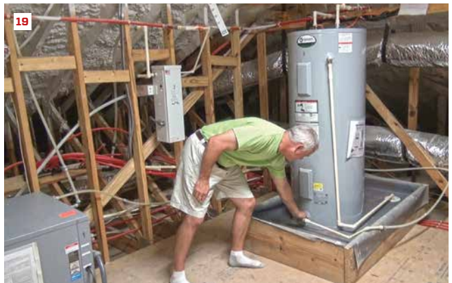
A preapplied paper ruler helps foam installers and inspectors verify application thickness (16). In this high-end system in an insulated attic, three zone supply ducts coming out of a distribution box are equipped with motor-controlled dampers (17); illuminated LEDs on the control device indicate which zones are active (18). Heat from the geothermal system also preheats hot water (19).
