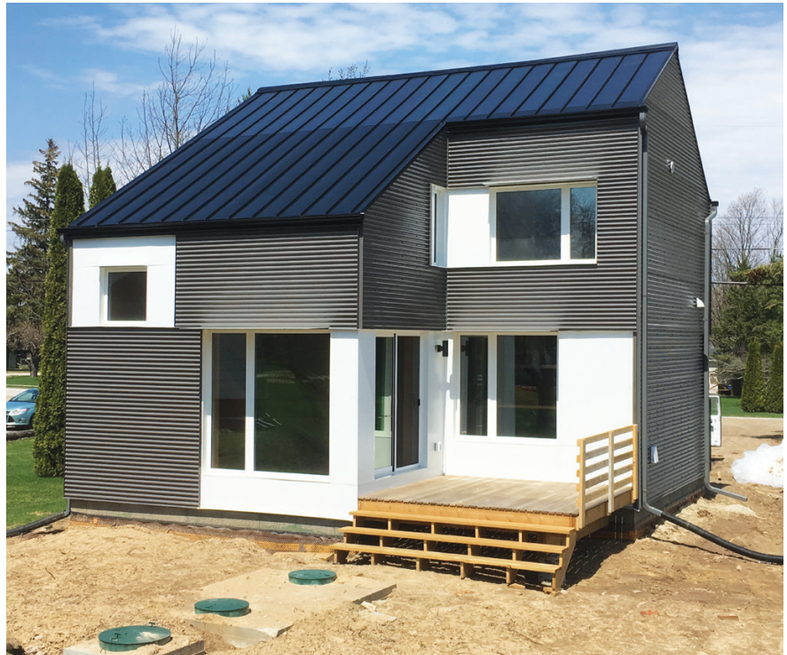
Built by Chris Magwood's Endeavour Centre in Clarksburg, Ont., this 1,100-square-foot zero-energy house cost $254 per square foot and stores 24 tons of CO 2 .
