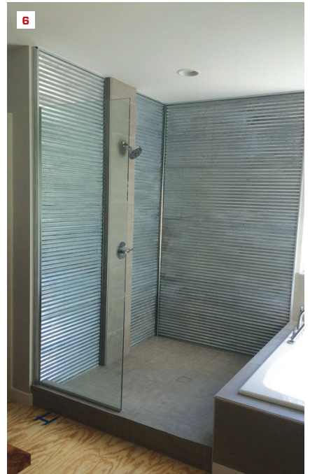
Finishing up. The central column stands proud of the metal panels. Once tiled, it provided a flat surface for the showerhead and mixer trims (4). At the corners of the tiled column, a reverse corner, using metal corner stock, echoes the detail used for outside corners on the exterior (5). In the finished shower, the metal panels create a brighter space and the desired industrial look (6).
