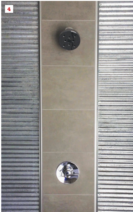
Finishing up. The central column stands proud of the metal panels. Once tiled, it provided a flat surface for the showerhead and mixer trims (4). At the corners of the tiled column, a reverse corner, using metal corner stock, echoes the detail used for outside corners on the exterior (5). In the finished shower, the metal panels create a brighter space and the desired industrial look (6).
