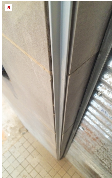
Finishing up. The central column stands proud of the metal panels. Once tiled, it provided a flat surface for the showerhead and mixer trims (4). At the corners of the tiled column, a reverse corner, using metal corner stock, echoes the detail used for outside corners on the exterior (5). In the finished shower, the metal panels create a brighter space and the desired industrial look (6).
