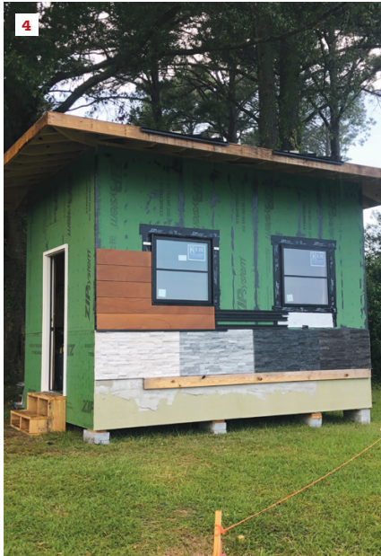
This small structure started out as a jobsite office (4) but soon became a perfect place to test different combinations of windows and claddings, including a thin adhered stone veneer in various colors and a rainscreen cladding system (5).
