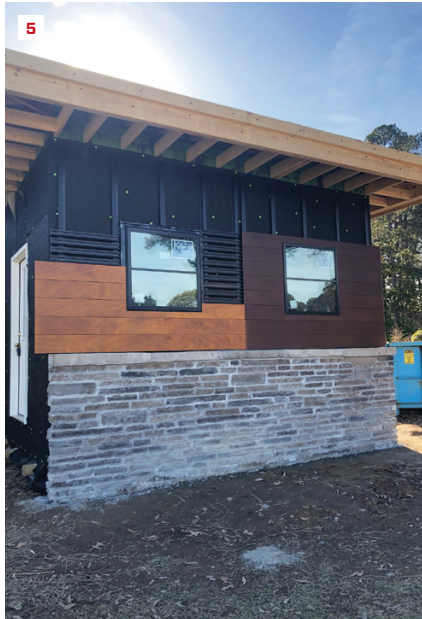
This small structure started out as a jobsite office (4) but soon became a perfect place to test different combinations of windows and claddings, including a thin adhered stone veneer in various colors and a rainscreen cladding system (5).
