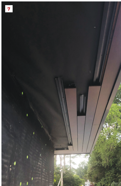
A full-scale mockup allows clients to visualize the difference between raked and full mortar joints in the stone cladding and the mitered Parklex cladding corner detail (6), and the effect of using a narrower, 4-inch version of the cladding for the soffit (7).
