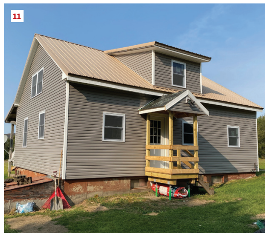
The replacement wall was pieced together from the inside out (7). The author worked his way down the rear wall (8), then the front bearing wall, and finished up with the gable end (9, 10). Although the home was clad with vinyl siding (11) and the exterior “essence” of the log cabin was removed, the main goals were to improve the comfort and longevity of the home.
