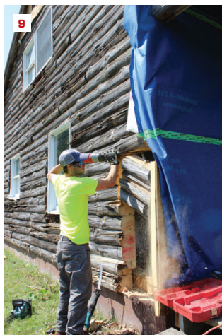
The replacement wall was pieced together from the inside out (7). The author worked his way down the rear wall (8), then the front bearing wall, and finished up with the gable end (9, 10). Although the home was clad with vinyl siding (11) and the exterior “essence” of the log cabin was removed, the main goals were to improve the comfort and longevity of the home.
