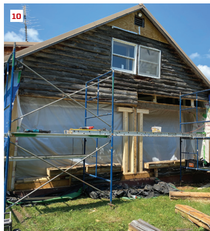
The replacement wall was pieced together from the inside out (7). The author worked his way down the rear wall (8), then the front bearing wall, and finished up with the gable end (9, 10). Although the home was clad with vinyl siding (11) and the exterior “essence” of the log cabin was removed, the main goals were to improve the comfort and longevity of the home.
