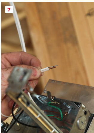
The author twists the green ground from the fixture with the bare conductor of the switch leg (5). Next, he strips about 1/2 inch of insulation from the white and black conductors of the switch leg (6), leaving the braided fixture wires longer than the solid switch-leg conductors (7). After twisting the conductors with wire nuts (8), he pushes the bundles into the box (9).
