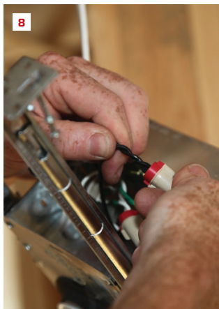
The author twists the green ground from the fixture with the bare conductor of the switch leg (5). Next, he strips about 1/2 inch of insulation from the white and black conductors of the switch leg (6), leaving the braided fixture wires longer than the solid switch-leg conductors (7). After twisting the conductors with wire nuts (8), he pushes the bundles into the box (9).
