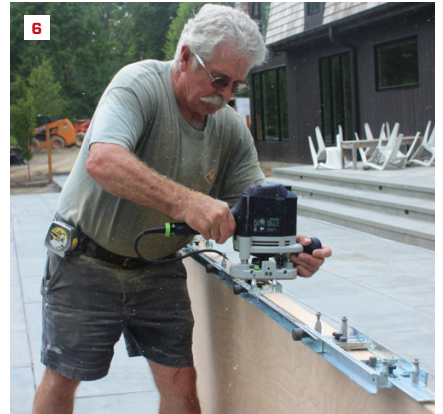
The head piece laps over the jambs (4). Ed Brady uses a multi-tool to notch out material on the head piece to create 1/2-inch returns, which will allow it to slip around the wall (5). After setting the door upright on its side in custom-built door stands, the author routs the hinge locations using a Porter-Cable hinge butt template kit (6).
