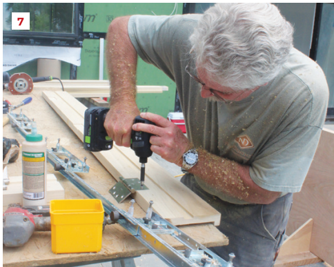
The author installs the door hinges on the routed hinge-side door frame (7) and fastens the frame to the door (8). Working inside, he and Brady position the door and frame assembly into place hands-free using a pair of Door Studs (9).
