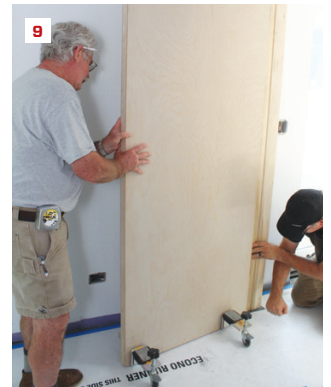
The author installs the door hinges on the routed hinge-side door frame (7) and fastens the frame to the door (8). Working inside, he and Brady position the door and frame assembly into place hands-free using a pair of Door Studs (9).
