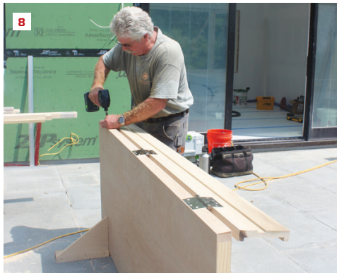
The author installs the door hinges on the routed hinge-side door frame (7) and fastens the frame to the door (8). Working inside, he and Brady position the door and frame assembly into place hands-free using a pair of Door Studs (9).
