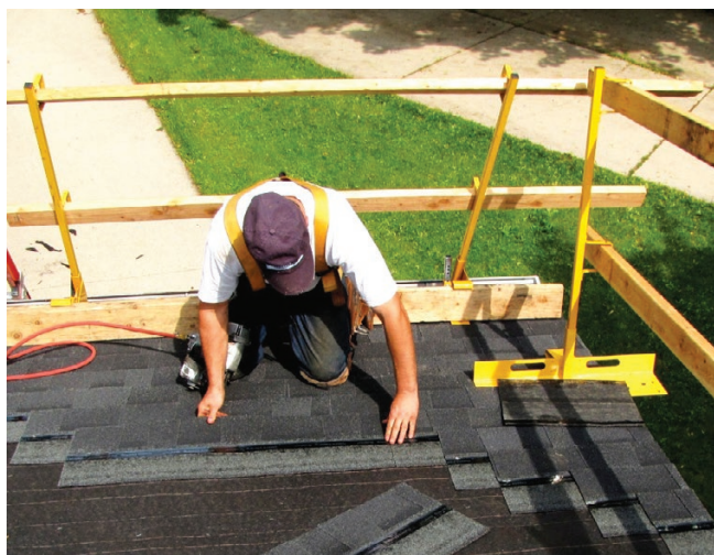
Fitted with guardrail holders, these roof brackets act as slide-guards and toe boards while providing fall protection.
