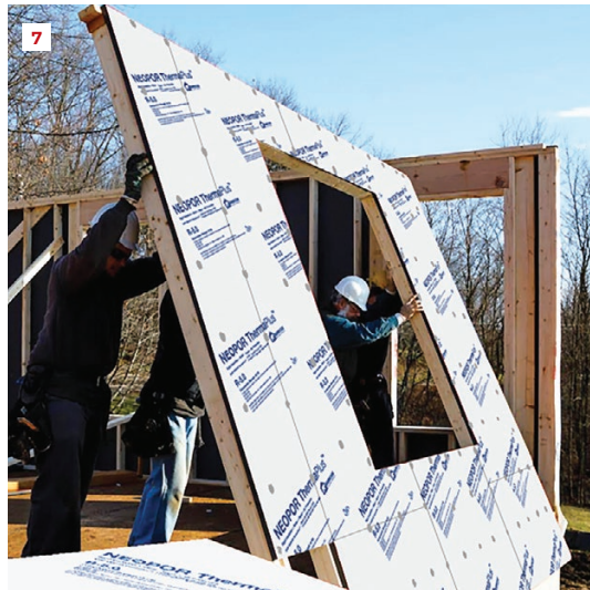
A range of low-carbon building materials: structural straw panels made by New Frameworks of Burlington, Vt. (6); Neopor low-carbon rigid foam panels from BASF (7); EcoCocon straw wall system from Build With Nature (8); hemp insulation from Nature Fibres (9).
