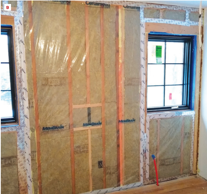
On this bedroom wall, which extends to the kitchen below, we used Certainteed's MemBrain, a material that allows water vapor to pass through when humidity levels are high while stopping airflow (9). The membrane worked well to reduce the amount of cooking odors that permeated into the bedroom.
