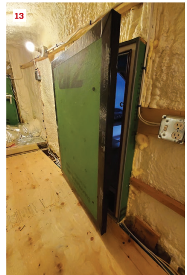
Access hatches from the exterior into a crawlspace (11) and from the interior into a knee-wall attic area (12, 13) are often leaky. For each one, we took care to build insulated access hatches with Zip System sheathing and foam-rubber gaskets.
