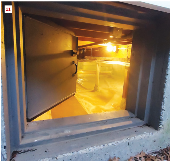
Access hatches from the exterior into a crawlspace (11) and from the interior into a knee-wall attic area (12, 13) are often leaky. For each one, we took care to build insulated access hatches with Zip System sheathing and foam-rubber gaskets.
