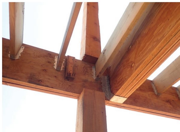
Figure 1. Discontinuous posts don't provide adequate resistance to uplift and lateral forces on a multilevel deck.
