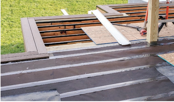
The PWT preservative-treated LVL framing has been flashed for additional protection.
