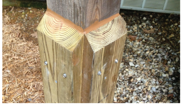
This UC4A-treated 6x6 southern pine post has been repaired using UC4B-treated 2x6 cleats and 1/4-inch-by-3-inch structural fasteners. Note that the cleats (as well as the concrete, not shown) have been sloped to shed water.
