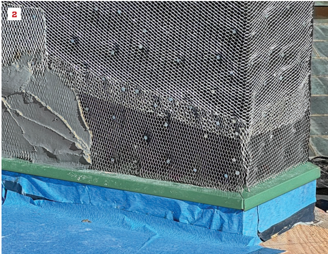
Both photos above (2, 3) show the through-flashing that is installed before the cladding. In each case, the author's company has installed a peel-and-stick roof underlayment first. Once the roofing and step flashings are installed, a second counterflashing will cover the step flashing and connect to this through-flashing.
