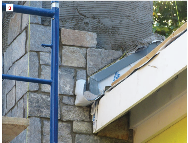
Both photos above (2, 3) show the through-flashing that is installed before the cladding. In each case, the author's company has installed a peel-and-stick roof underlayment first. Once the roofing and step flashings are installed, a second counterflashing will cover the step flashing and connect to this through-flashing.
