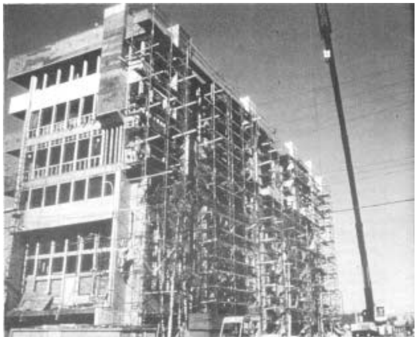
The Barrow Street Building under construction
