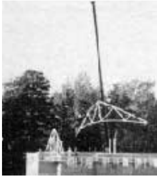
Figure 1. Pick trusses up from two points, not from the peak. Reason: Unbraced trusses are unstable and easily damaged under their own weight.
